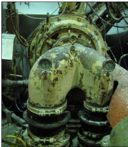
Figure 10: 2-zone couch and vacuum manifold
