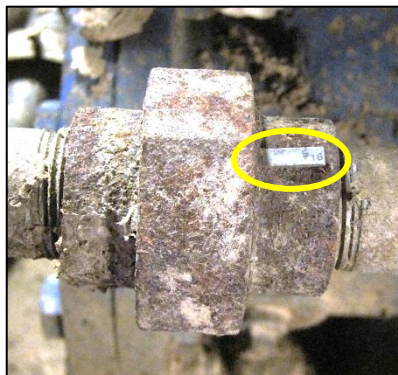
Seal water orifice union – note s/s tab
