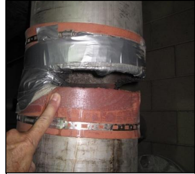
10" diameter vacuum line with failed rubber boot. Leak caused 5" Hg of vacuum reduction. Duct tape indicates previous attempt to fix.
