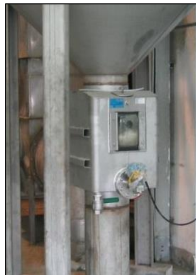
Ecoflow™ for measurement of uhle box and press nip flows
